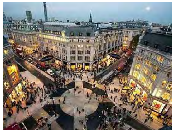
Junction improvements at Oxford Street/Regents Street, London
